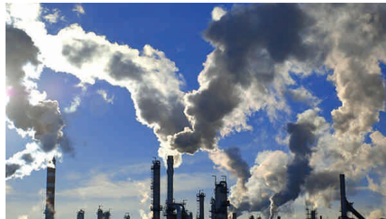
Cement plant flue gas desulfurization and denitration
