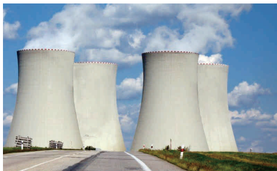
Power plant flue gas desulfurization and denitration
